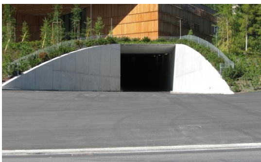
Tunnel to the supplier entrance
