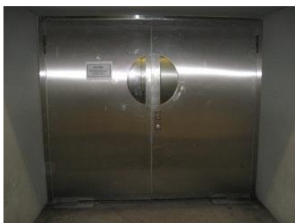
Front delivery section entrance, Building A
